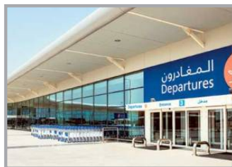
Dubai World Central International Airport- Passenger Terminal
