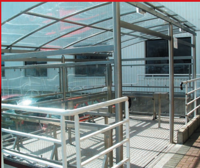
Stainless steel smoking booth built to requirements , complete wit stainless steel seating, stainless steel ashtrays and stainless steel catch bins.
